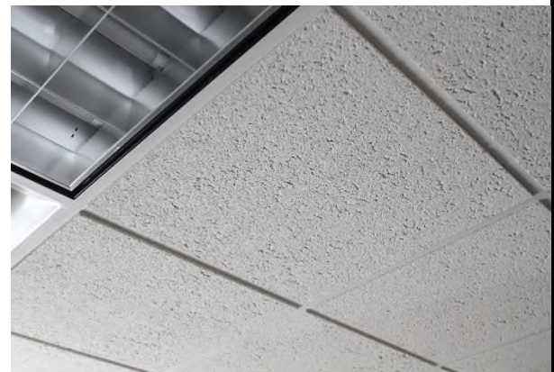
24. Sample 23 , Second Floor – S/W Copier, 2x2 Ceiling Tile, White.
