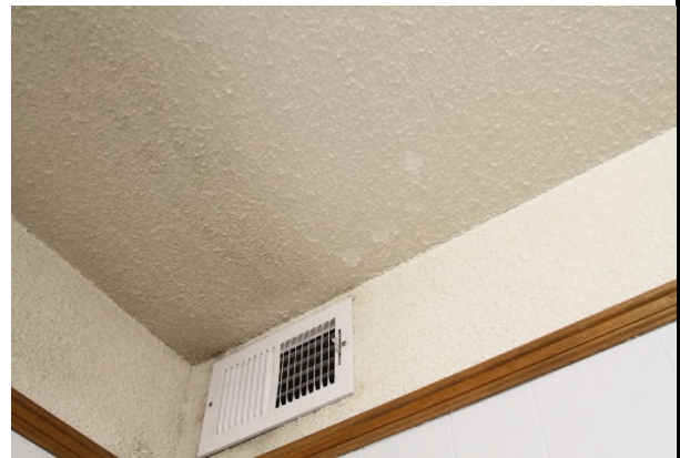
28. Sample 27 , Second Floor – Open Office, Textured Ceiling.
