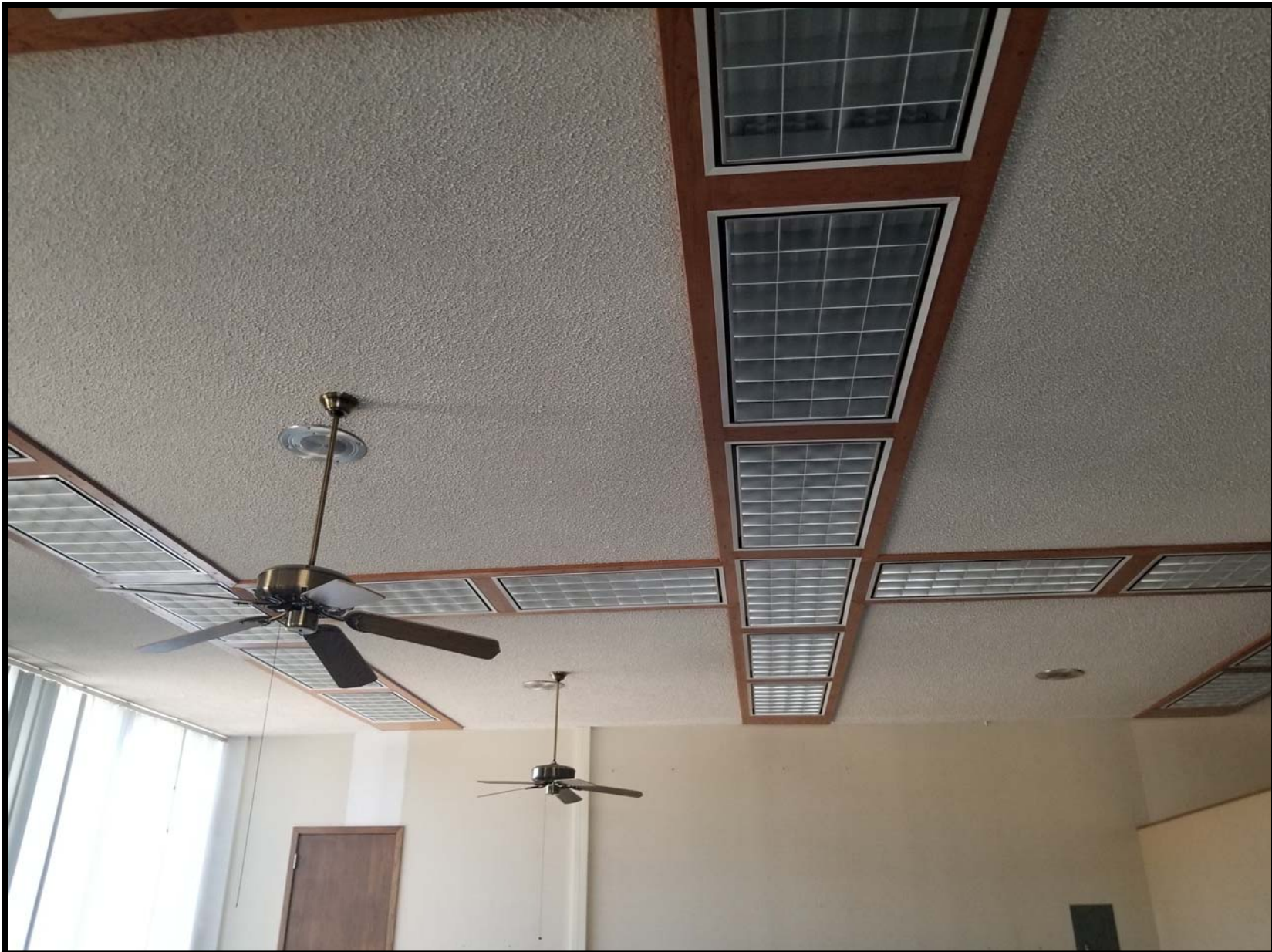
Photo FF9 - Looking easterly from the northwest offices on first floor.
