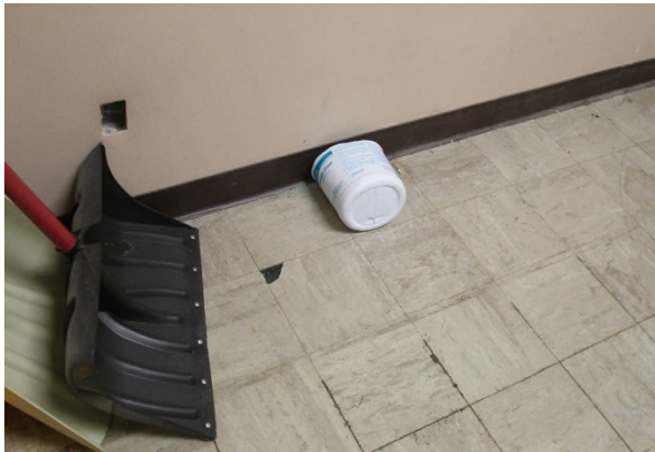
21. Sample 20 , First Floor – Drive Thru Vault, 9x9 VFT, Gray/Green w/Black Mastic.
