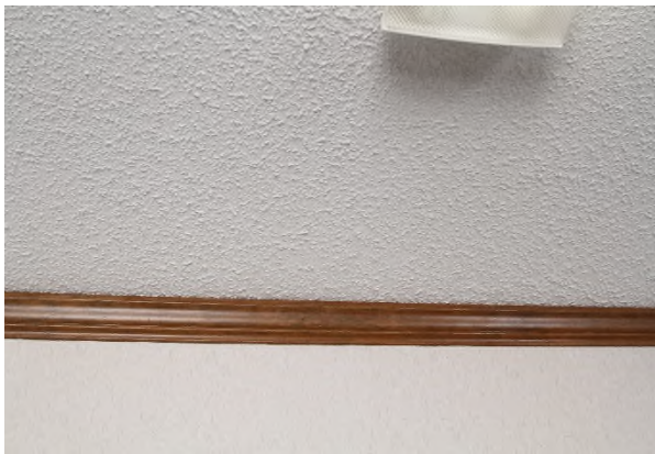
27. Sample 26 , Second Floor – East N/S Hallway, Textured Ceiling.
