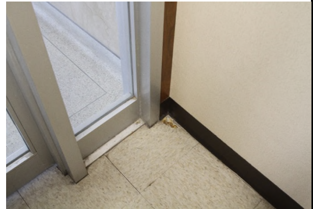
22. Sample 21 , First Floor – Council Lobby, 12x12 VFT, White w/Yellow Mastic.
