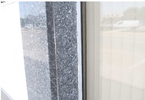
23. Sample 22 , First Floor – Exterior Window, Window Glazing, Gray.
